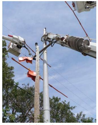
Replacing an end of useful service life wood pole with a ductile iron pole.
